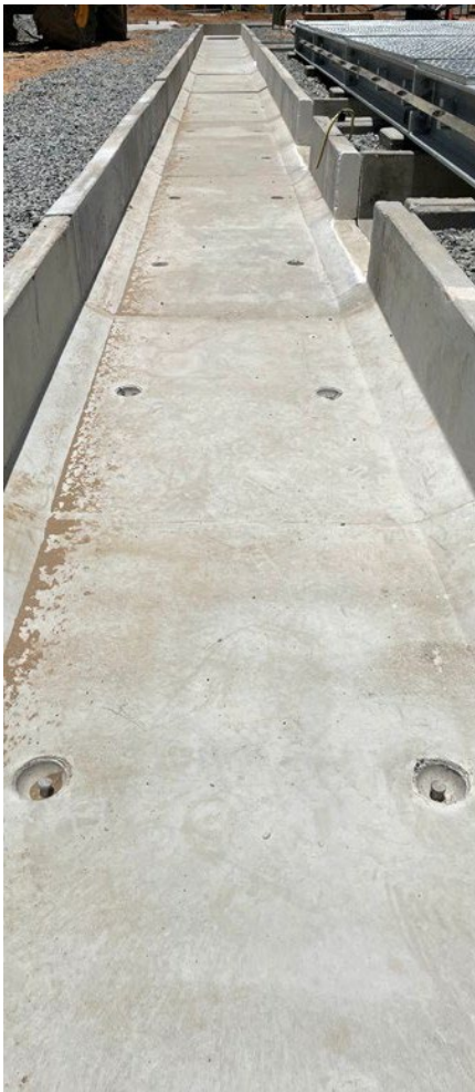
Concrete Cable Duct
